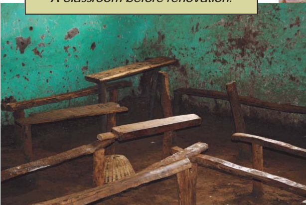
A classroom before renovation.
