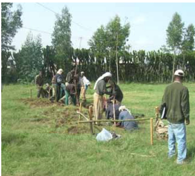
Parents digging the school foundation
