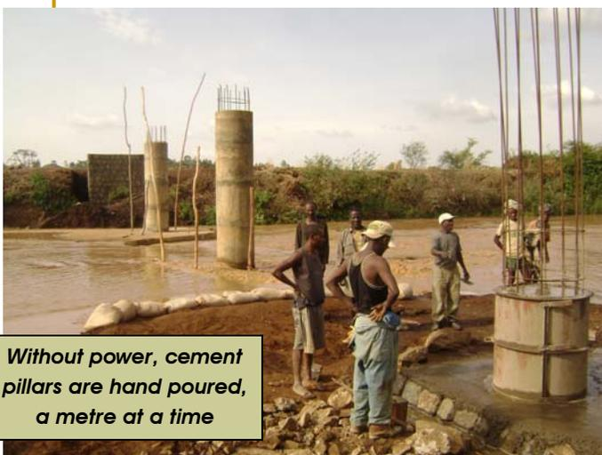
*Without power, cement pillars are hand poured, a metre at a time*
